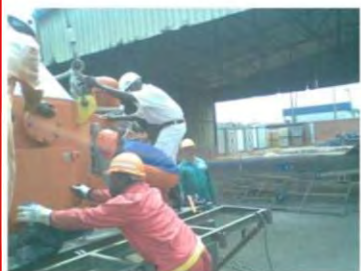
Handling and presentation of the centrifuge on the fabricated platform
