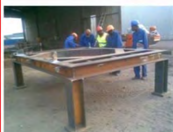
Platform fabrication on SOMAINTO Sarl Site
