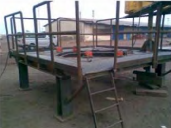
A view of the Platform completed before Sanding & Painting
