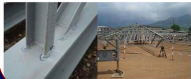
QUALITY CONTROL OF ROOF TANK STRUCTURE
